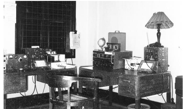
The new transmitter and its BC221, VFO AR88 and spare BC-221
